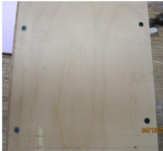
Photo #14: Roof screwed onto bee house.
