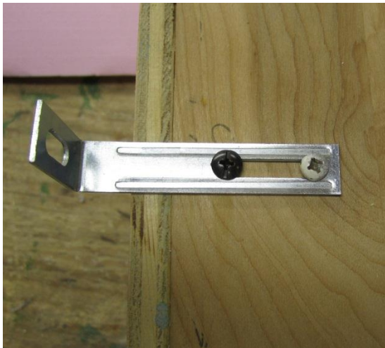
Photo #15: Mounting bracket attached to side of house.
