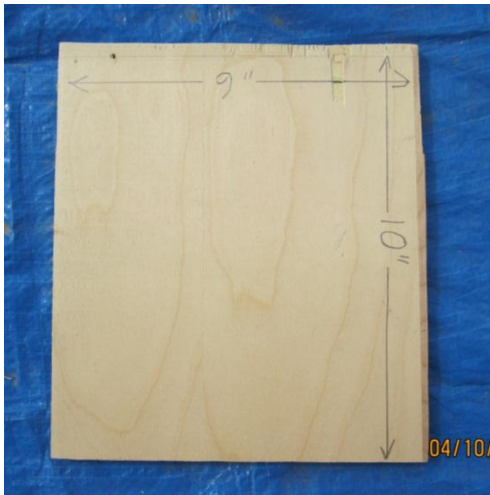
Photo #13: 9"x10" roof cut out.
